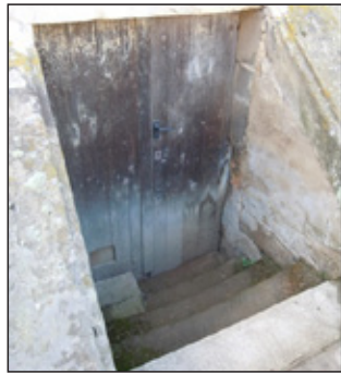
Door to cellar
