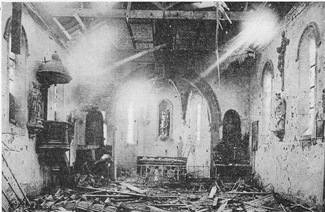
Interior of Church at Cunel.
