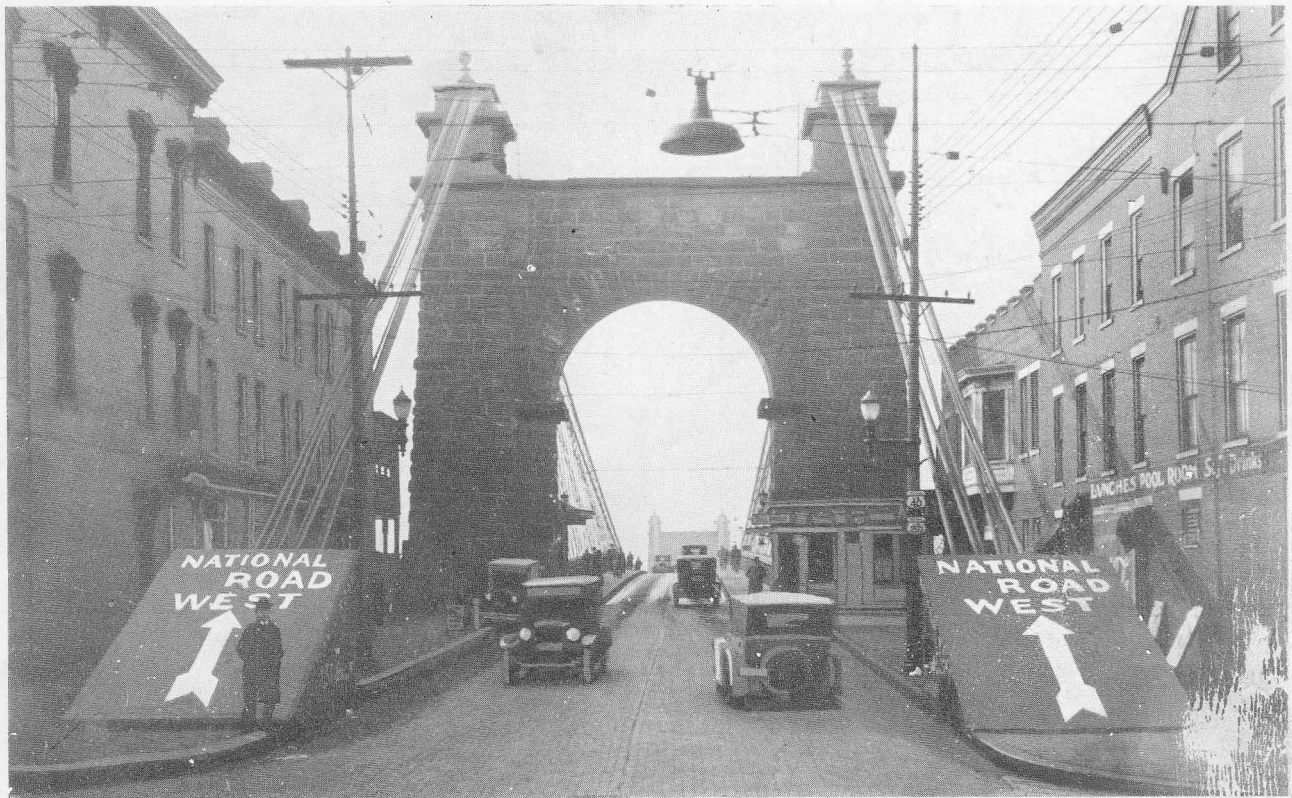
The suspension bridge at Wheeling, West Virginia, built in 1849, which until the completion of the Brooklyn Bridge, was the longest suspension bridge in the new world.
