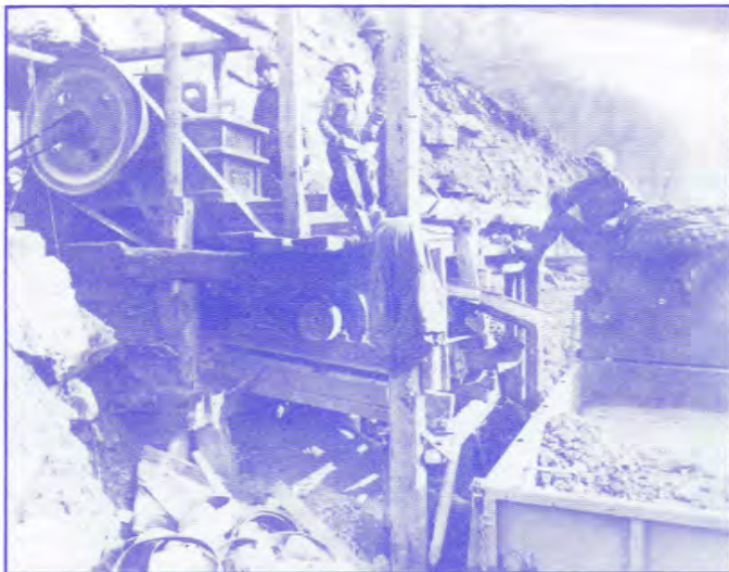
Men of 305 Engr Bn, 80 Div. use a German rock crusher to make road fill near Crutchen, Germany. February 20, 1945
